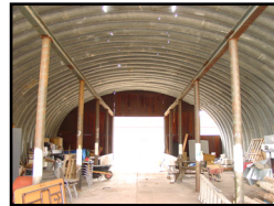
The steel frame in the existing building will be salvaged for use in the new building.
