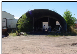
Existing storage structure to be dismantled and the new technology center will be built in its place.
